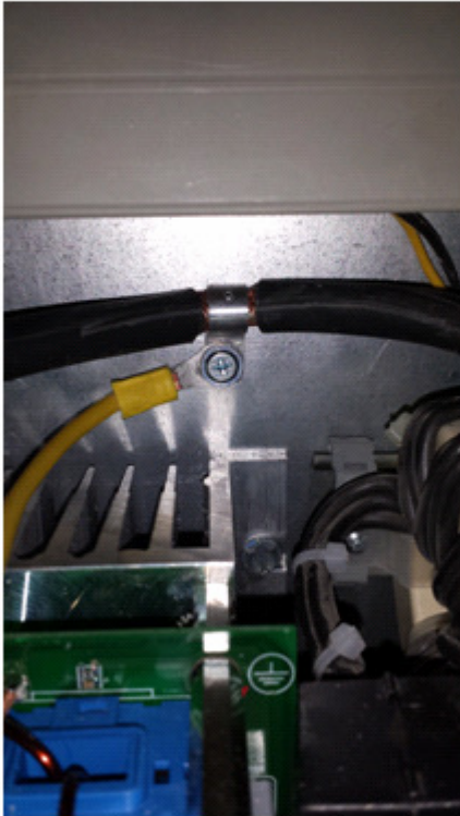
Correct earth termination for brake resistor
